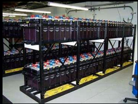
Batteries tests benches
